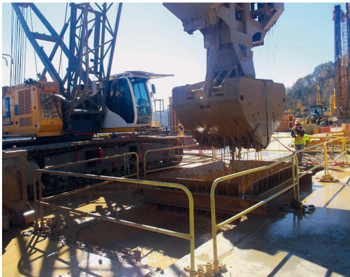
Figure 6. MC96 with hydraulic grab
