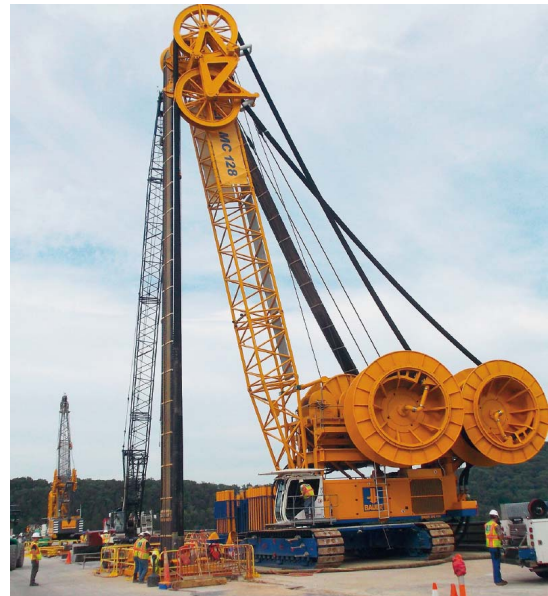
Figure 7. MC128 with BC50 cutter
