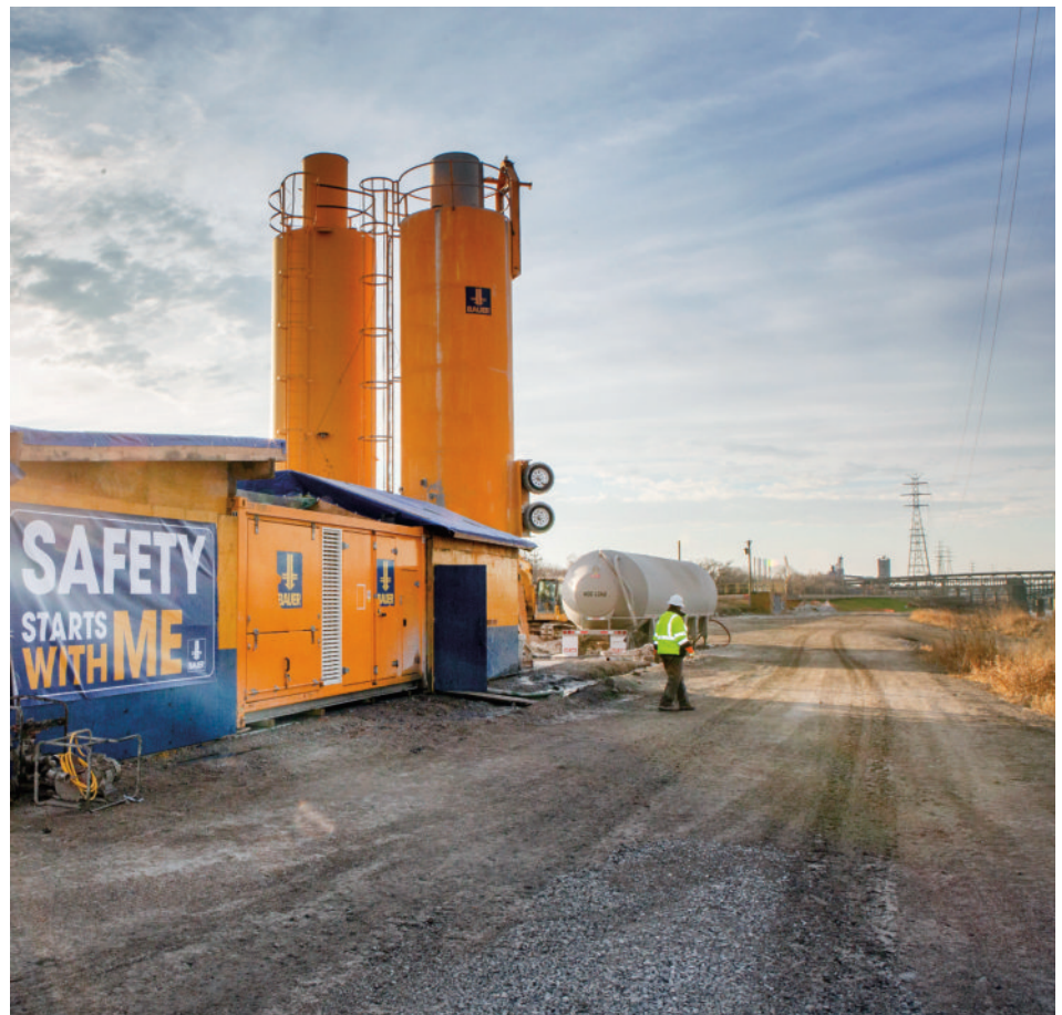
Jet grouting plant
