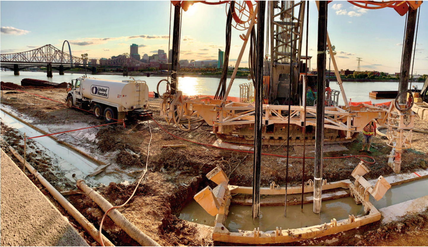
Completed panel excavation at the downstream end of the project
