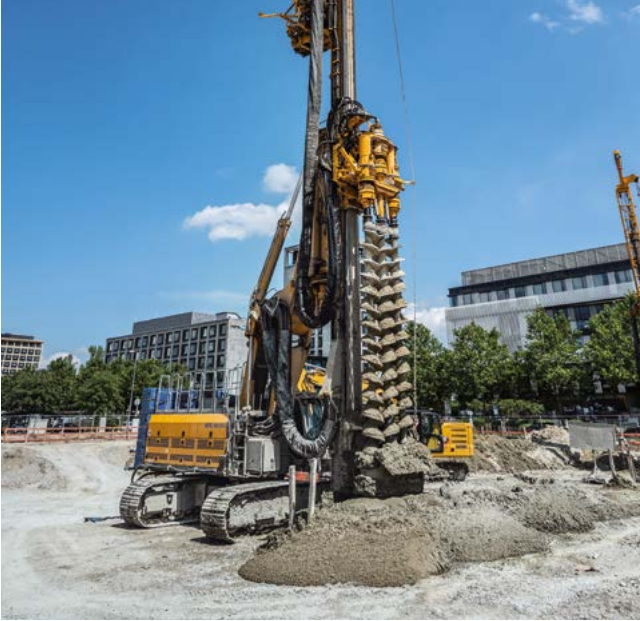
Parkstadt Schwabing, Munich, Germany Construction of a 6,000 m 2 single-anchored Mixed-in-Place cut-off wall for a 9 m deep excavation pit.
