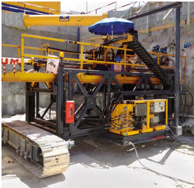
Pedestrian tunnel, Doha, Qatar Controlled drilling for sealing and stabilizing injection in a 90-m pedestrian tunnel.
