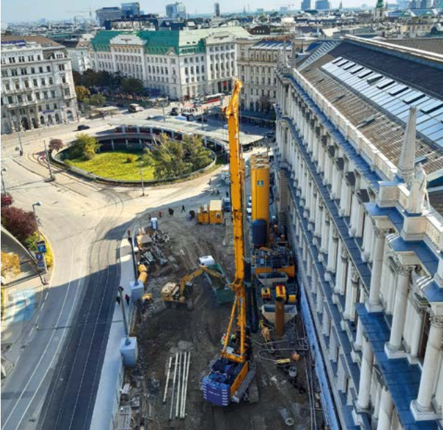
Subway line crossing, Vienna, Austria Construction of roughly 35,000 m of bored piles with varying diameters of up to 1,180 mm and drilling depths of up to 61 m.
