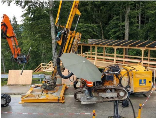
Rosshaupten Dam, Germany Installation of a rock grouting curtain up to a maximum depth of 91 m.
