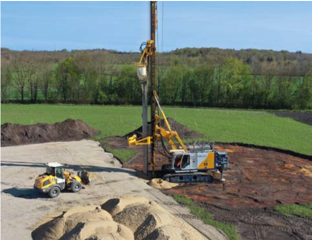
Wind park, Silberstedt, Germany For the foundation of several wind turbines, a total of 3,200 m of vibration replacement were carried out.
