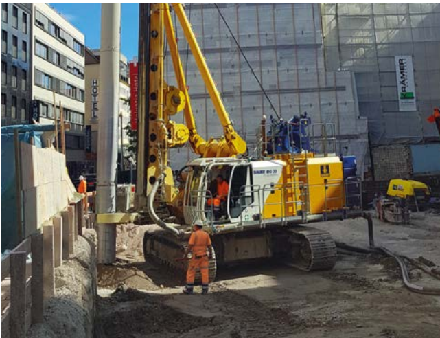
New construction of office building, Munich, Germany Execution of secant pile wall with a diameter of 620 mm and depth of 18 m using the FoW method.
